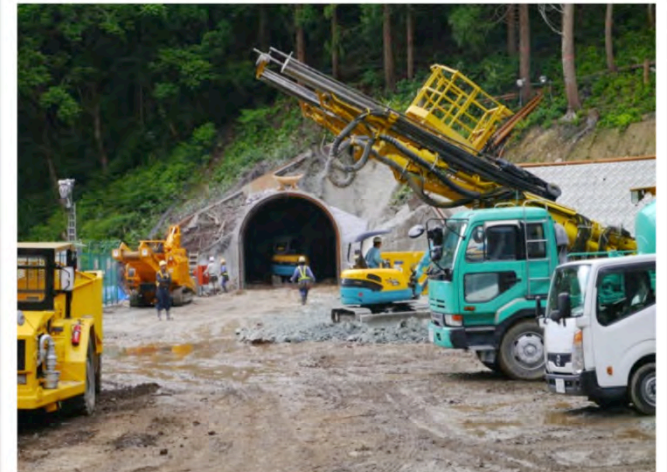
Tunnel excavation (main entrance to the experimental area)
