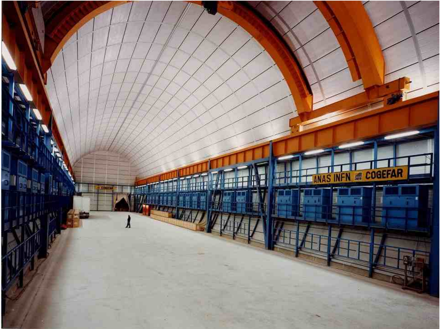
Hall B after construction
