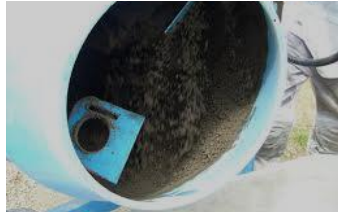
Preparation of mortar
